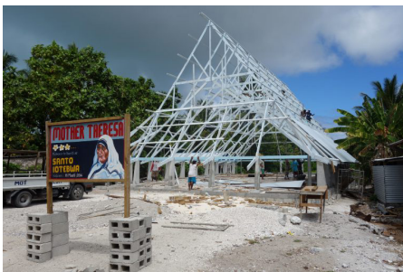
A manebaba being built with non-traditional framing, Temaiku
